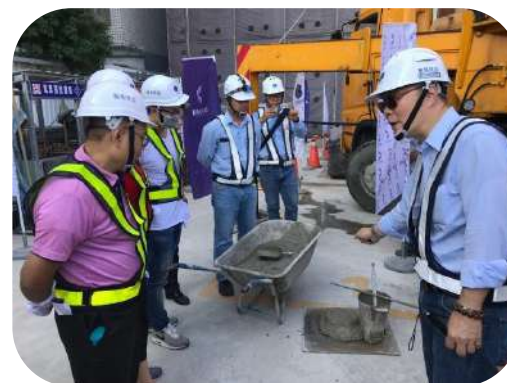
混凝土坍度實驗
