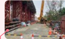
Surrounding pipe of construction equipment working area (turning radius)
