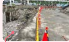
Construction work area partition warning line
