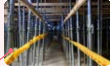
Set up secure channels in construction areas
