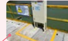
Drawing-line management in the temporary electrical panel placement area
