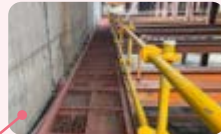
Set up secure channels above the strutting
