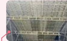
The safety net is fully paved under the falsework
