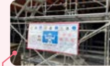
Construction frame inspection and assignment of qualified work supervisors
